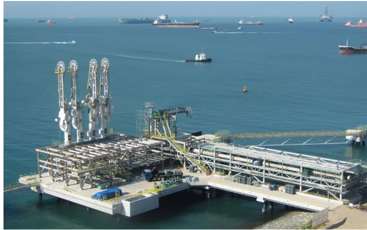
Gambar 1. 5 Instalasi Pipe Rack Di Dermaga Sumber : Google Image
