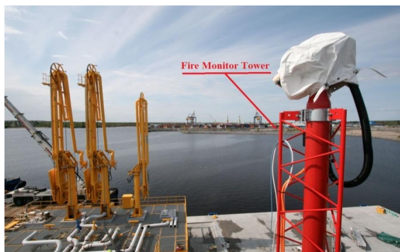
Gambar 2. 24 Fire Monitor Tower
