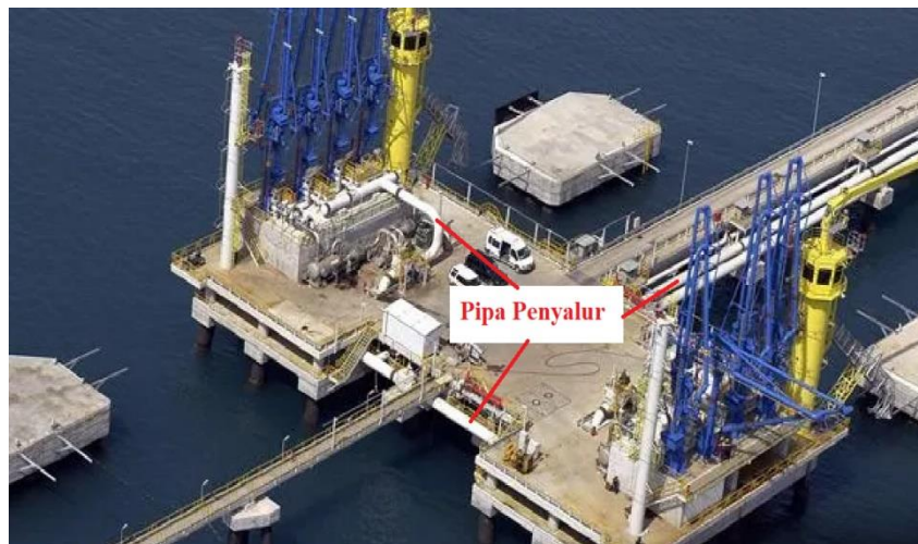
Gambar 2. 23 Instalasi Pipa Jetty Head
