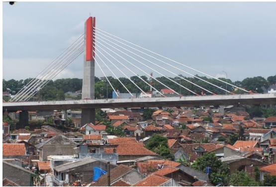
Gambar 2. 19 Jembatan tipe kabel ( cable stayed )
